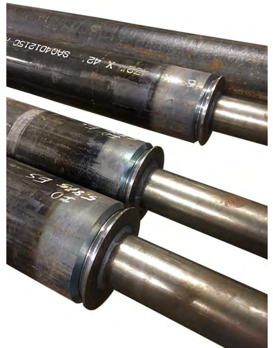
Pipe is Carefully Heated and Shafts Inserted to Specified Depth
